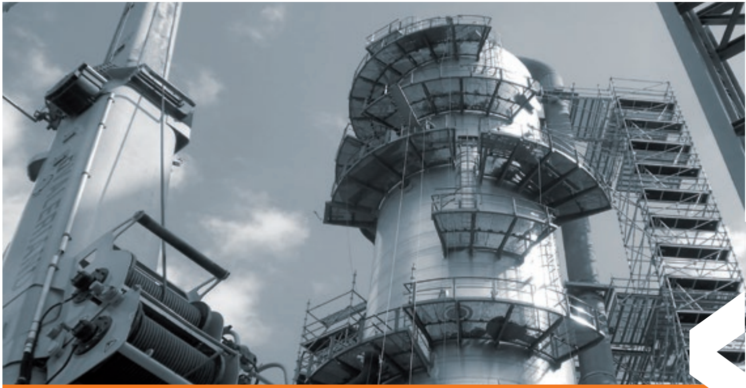
Europoort Power Plant in the Netherlands. The multidirectional RINGSCAFF system was ideal for the work on the power plant in Rotterdam. Thanks to its flexibility, the scaffolding could be adapted to the challenging shape of the object.
