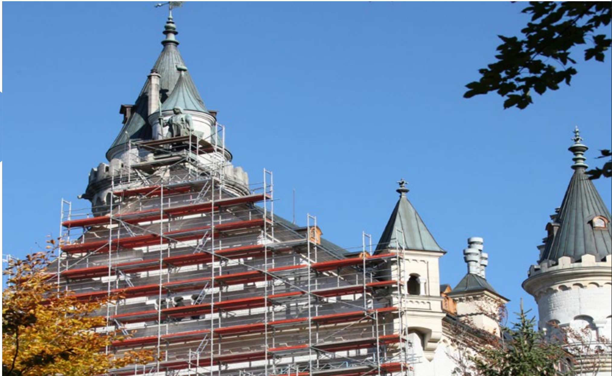
Castle Neuschwanstein in Germany. Narrow access roads, impassable terrain and crowds of visitors notwithstanding, Scafom-rux SUPER 65 scaffolding system in combination with a modular scaffolding system was erected to renovate the exterior façade of the globally known historic building.
