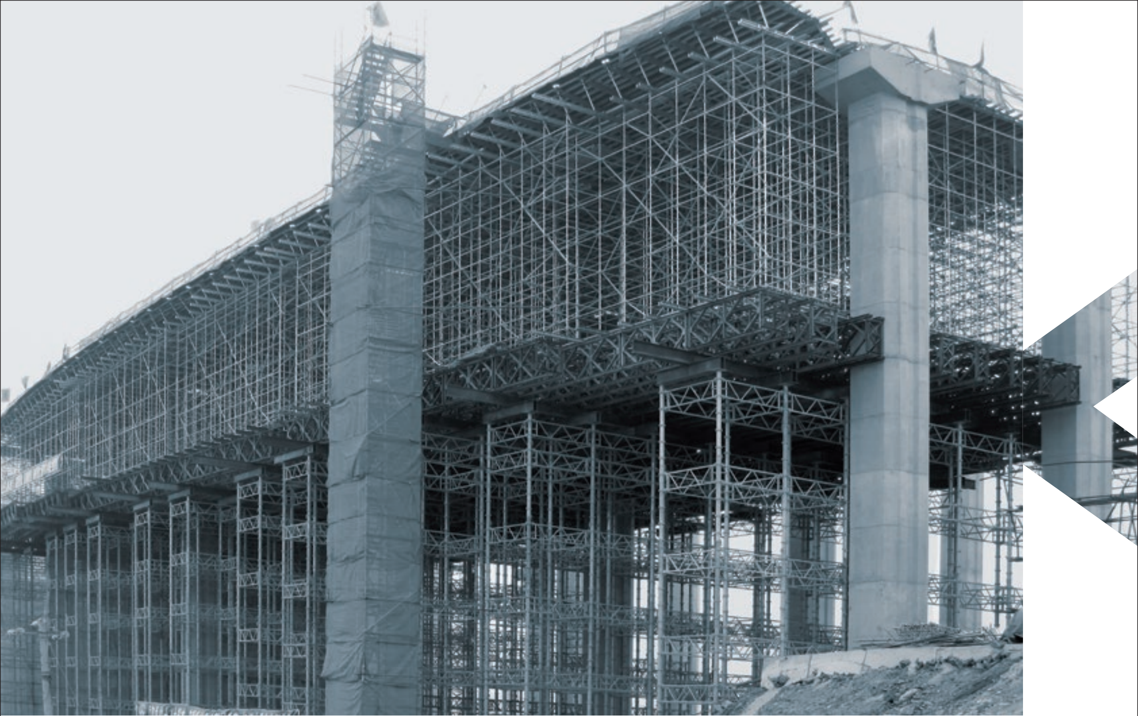
Guilong Highway in China. One million cubic metres of SPS, Duralok and SBS 135 material were used for the construction of the 12 km long Highway in the Guizhou Province. Special designs of shoring had to be done for the project.
